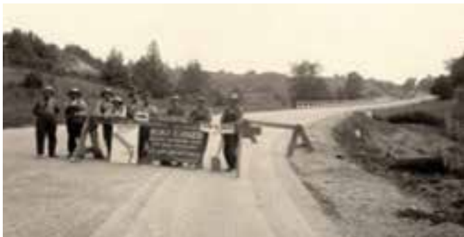
Construction on Highway 11, July 1924, near Holland Landing
